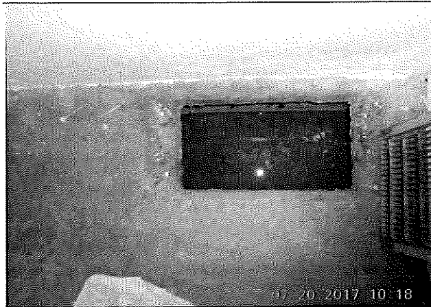
VIEW OF RETURN AIR SYSTEM BELOW GRADE AFFECTED WITH PONDING WATER
