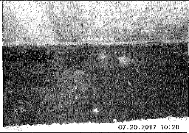
VIEW OF RETURN AIR SYSTEM BELOW GRADE AFFECTED WITH PONDING WATER
